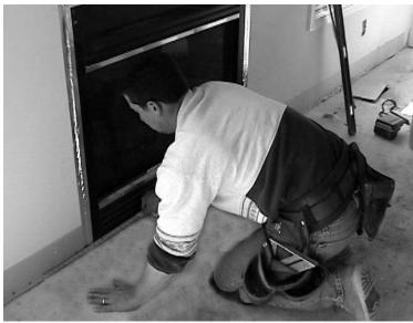
Measure and mark off the area around the firebox to determine where the hearth is going to fit on center. Apply several half dollar sized applications of silicone to the back of the hearth or floor where the hearth will rest. Silicone should be applied liberally, using enough to keep the hearth in place after silicone dries.
