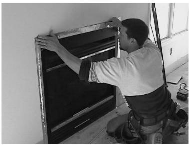
(Optional step.) In regions with extreme temperature variations adding an additional thermal barrier is recommended. With aluminum duct tape, tape around the firebox sealing the opening between the drywall and the firebox. (Available at local hardware stores.)
