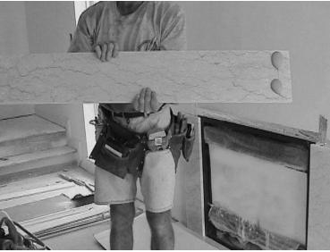
Apply silicone adhesive in 4 places (two at each end) to the back of the header at its outer ends and set it on top of legs. Pull back for 30 seconds and reposition header.
