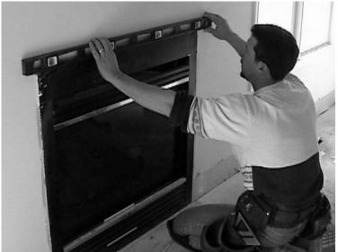
Ensure the fireplace is installed plumb and level. The face flushes with the outer surface of the wall. Correct any problems before proceeding. (It is a good practice to inspect the top of the firebox for trash or other combustible materials and remove them.)
