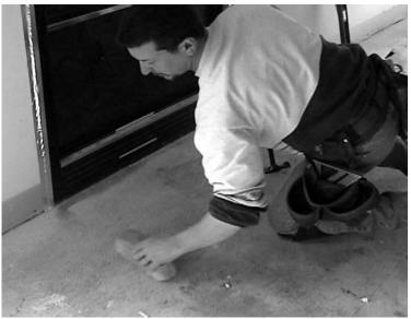
Make sure that the floor area in front of the fireplace is level and clean, and has minimal flex. Make sure there are no nail or screw heads protruding above the floor surface, if so take a hammer or drill and drive them in below the surface. (For wood-burning applications, a thermal break will need to be laid prior to hearth installation. "Micor" or "Wonder board" is recommended. See fireplace manufacturers recommendations.
