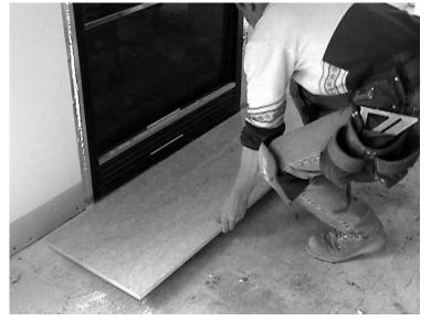
Lay hearth. For faster silicone set up, lift the hearth up from the floor and allow the silicone to "string" Wait 30 seconds and reposition the hearth.
