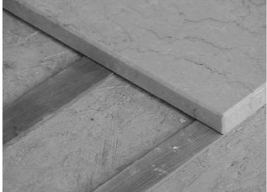
Once the hearth is in place check and make sure it is level. You may need to shim the hearth to get it level if the floor is uneven. Cut off excess shim. Caulk around perimeter of the hearth to support the edge where any gaps may be.
