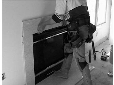
Push firmly against the wall, and make sure that everything is adjusted, as you want it. If needed you can shim behind the legs or header to create a flush joint between them. These can be removed or cut after the silicone dries. The shim will also help prevent the stone from moving. You may want to use a few pieces of aluminum duct tape, to ensure that legs and header stay in position until the silicone dries. (It may be necessary to build a wooden support to hold header in place.)
