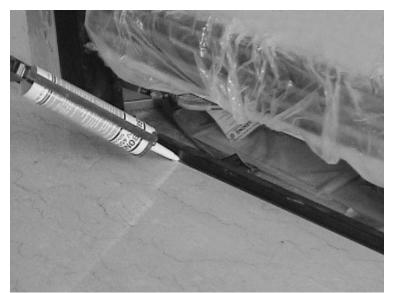
Check with local building codes as it may be necessary to caulk the inside front bottom edge with clear or black silicone. **Note:** this is required on wood burners.
